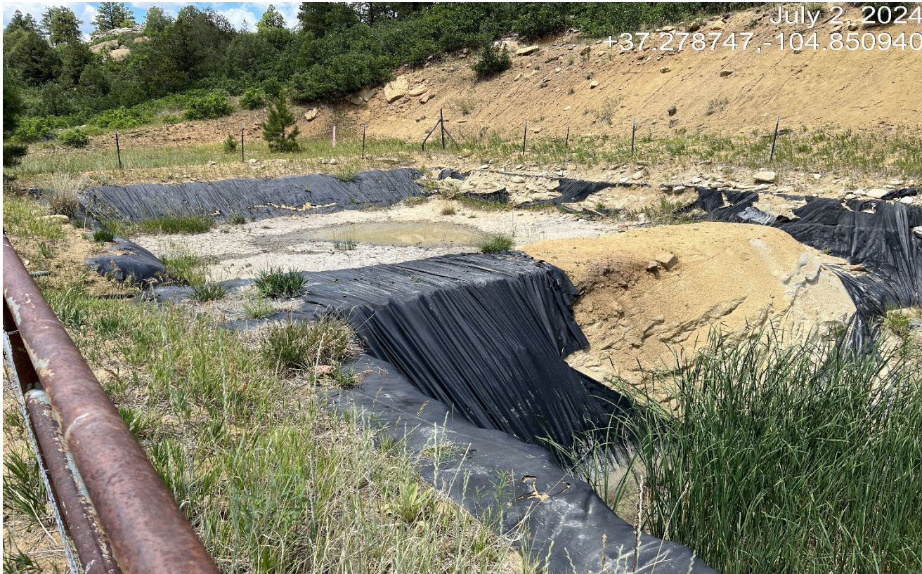
Photo 2. Facing toward the produced water pit. The liner is torn and degraded. There is grey drilling mud in the upper pit that needs to be cleaned out and removed. A form 27 will need to be submitted due to compromised pit.
