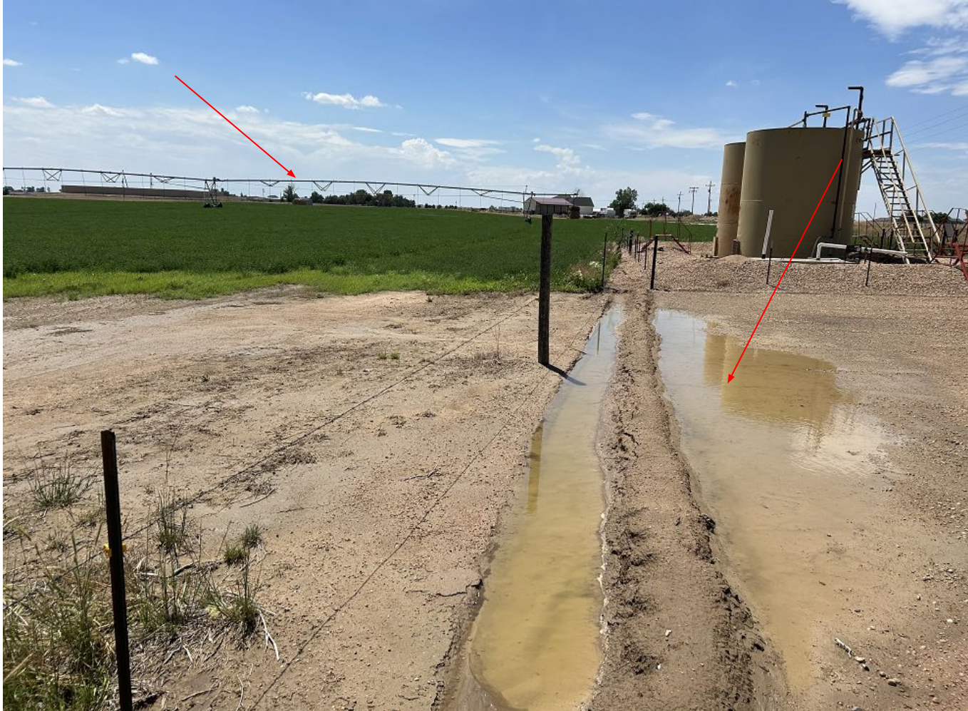
Photo 3. The photo is an Operator provided photo demonstrating the Operator has attempted to slow erosion on the tank battery location with a small berm. However the pivot seen in the background is causing ponding on the tank battery due to installed BMP's.
