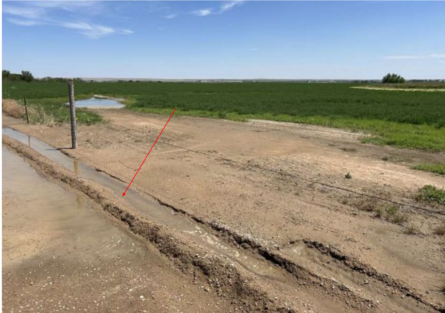
Photo 2. The photo is an Operator photo from FIRR #403838786 demonstrating the Operator has attempted to slow erosion on the tank battery location with a small berm.
