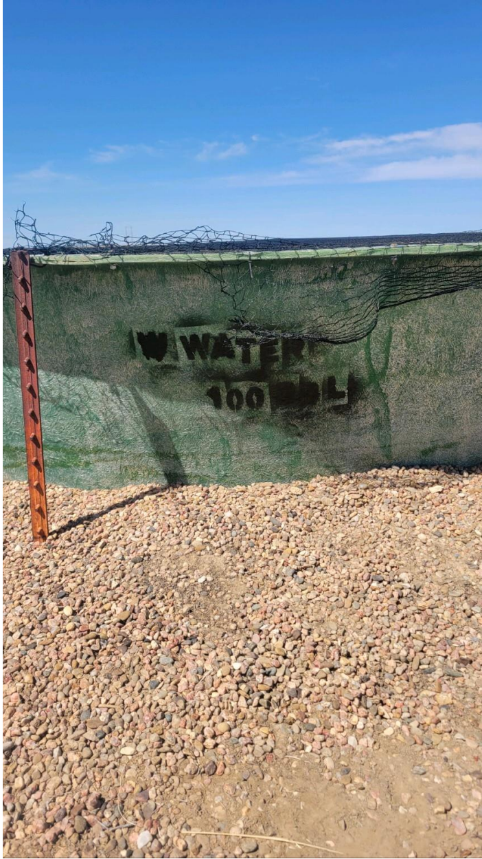
New netting installed. Berms were repaired. Volume of the tank stenciled on the tank.
