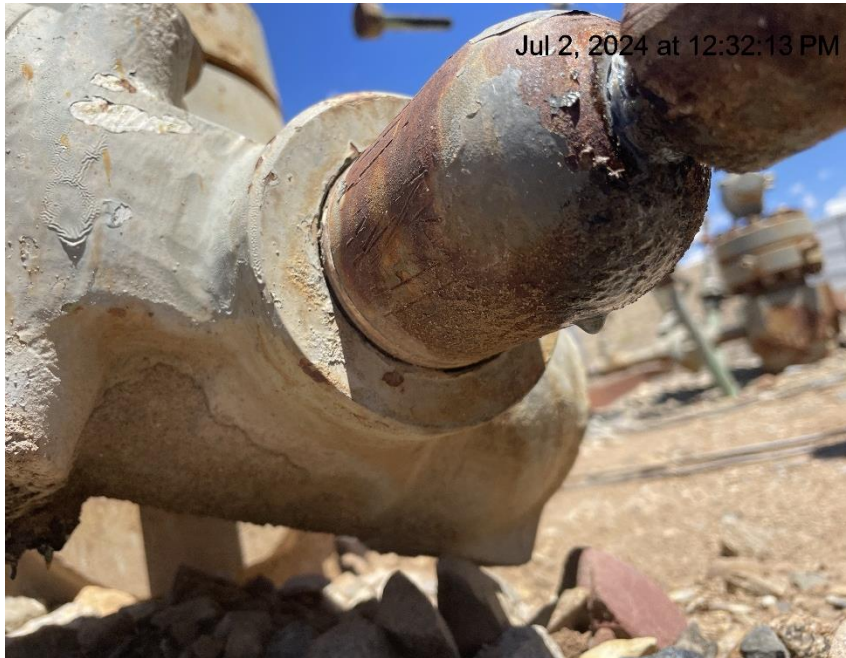
Photo # 2227 Mechanical Condition – possible leak on bullplug connected to RWF 432-26 well casing valve
