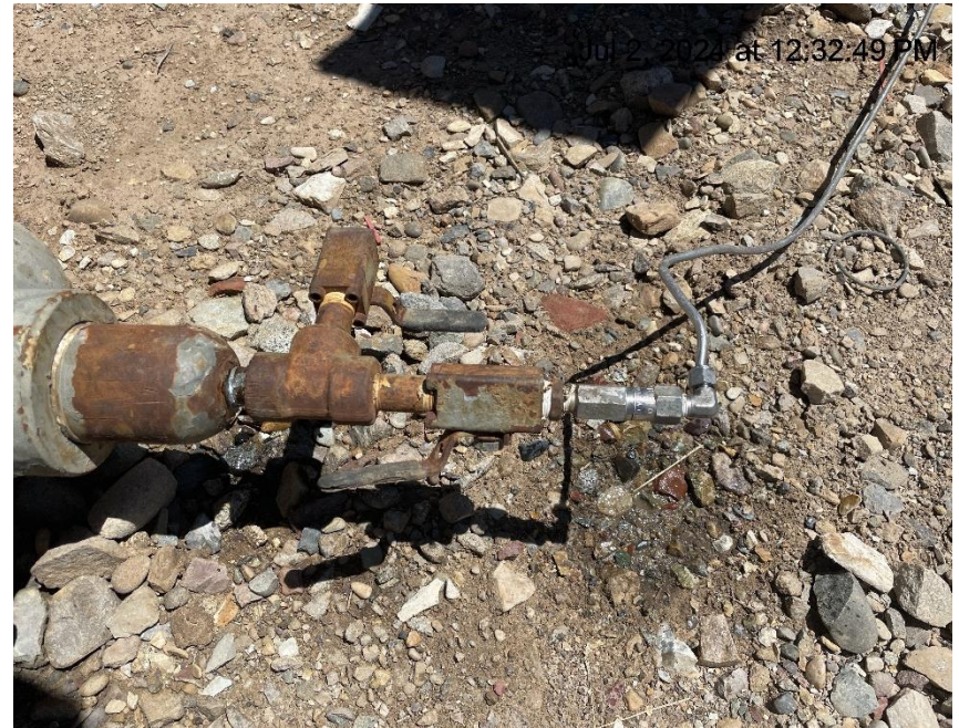
Photo # 2228 Mechanical Condition – possible leaks on chemical line & bullplug connected to RWF 432-26 well casing valve
