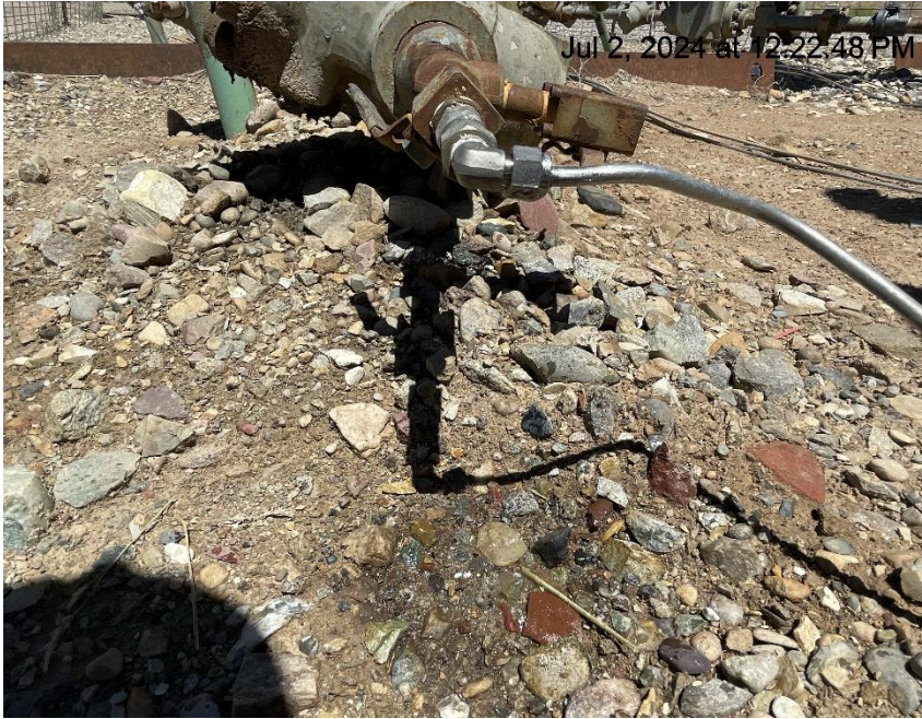
Photo # 2219 Mechanical Condition – possible leak on chemical line connected to RWF 432-26 well casing valve
