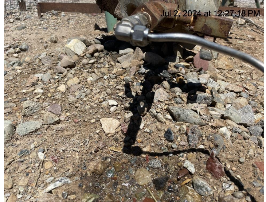
Photo # 2224 Mechanical Condition – possible leak on chemical line connected to RWF 432-26 well casing valve
