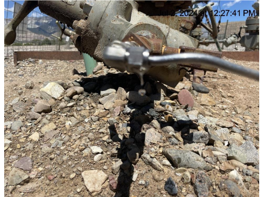
Photo # 2222 Mechanical Condition – possible leak on chemical line connected to RWF 432-26 well casing valve
