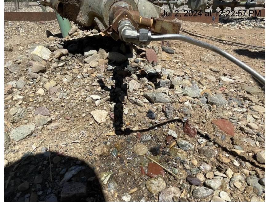
Photo # 2220 Mechanical Condition – possible leak on chemical line connected to RWF 432-26 well casing valve
