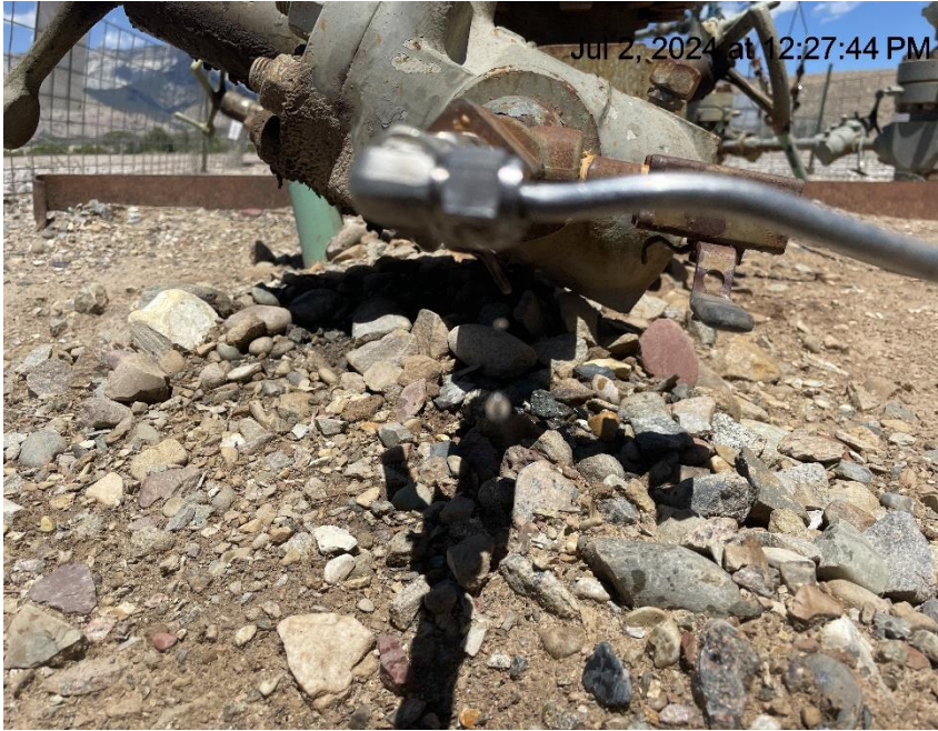
Photo # 2223 Mechanical Condition – possible leak on chemical line connected to RWF 432-26 well casing valve
