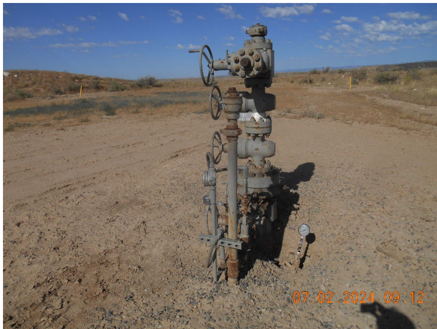
Wellhead during Bradenhead test
