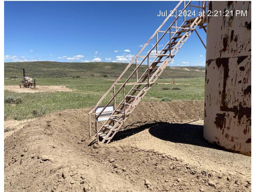
Location from Northwest corner
