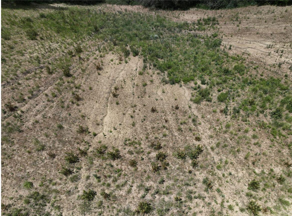
**Photo 10:** Aerial image showing areas on the west end of the Location where stormwater issues were observed. Erosion degradation observed throughout the slopes of the Location.
