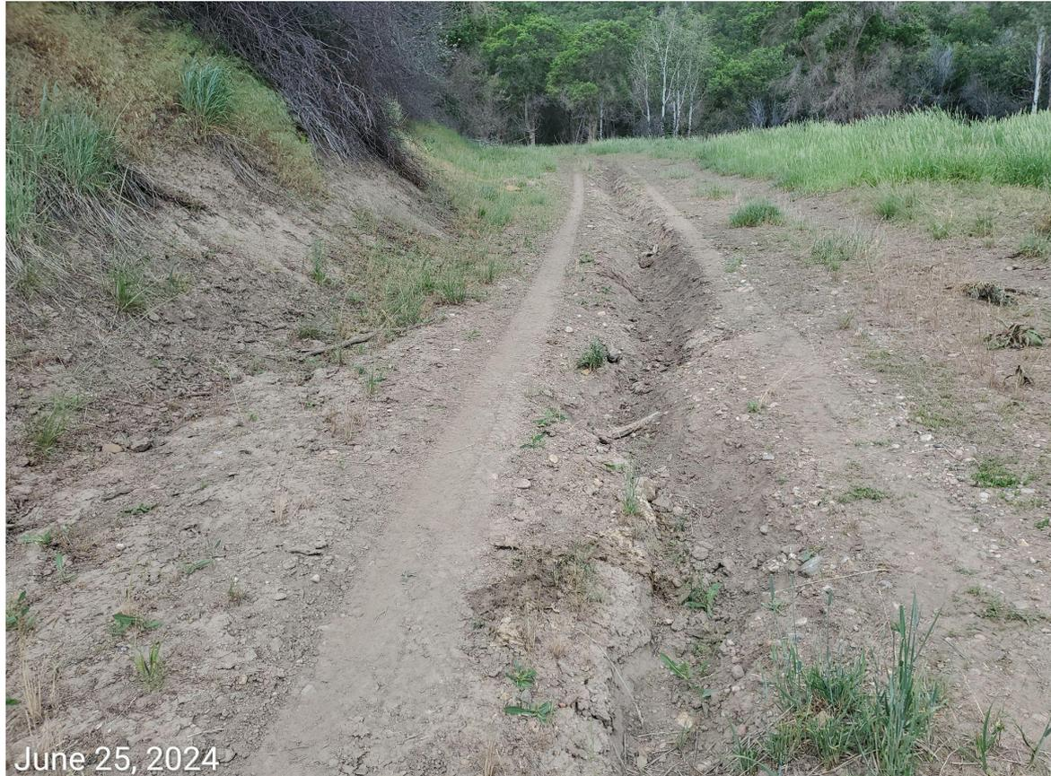
**Photo 11:** Photo taken from the access road. Photo examples showing erosion degradation issues observed on the road.
