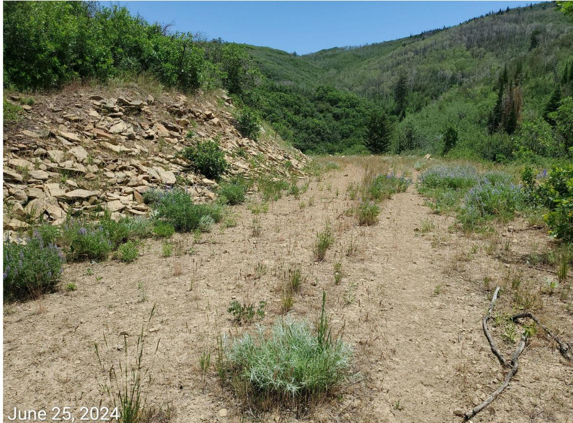
**Photo 4:** Photo example showing access road has not been recontoured/regraded and reclaimed in accordance with 1004 Rules.
