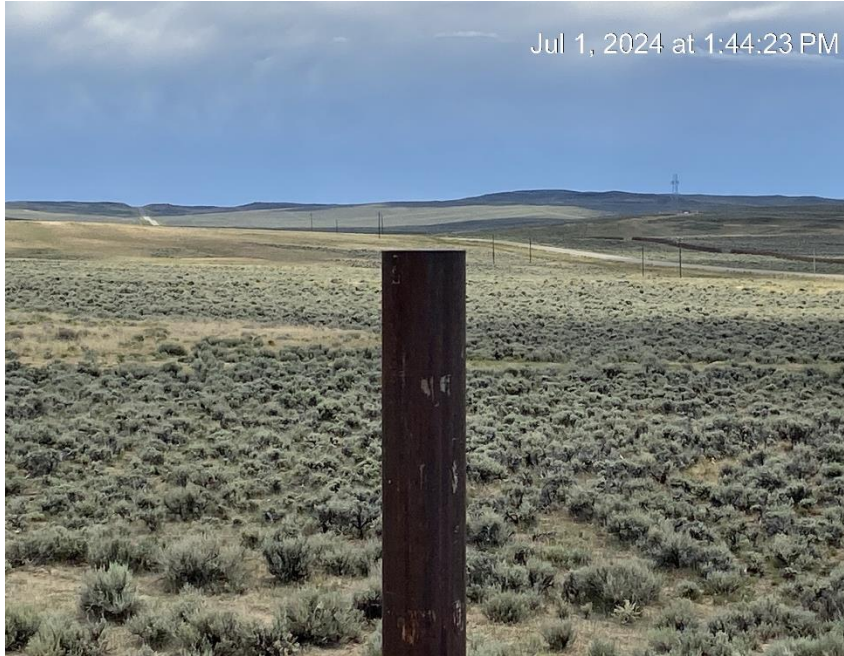
Vent riser missing wildlife protection
