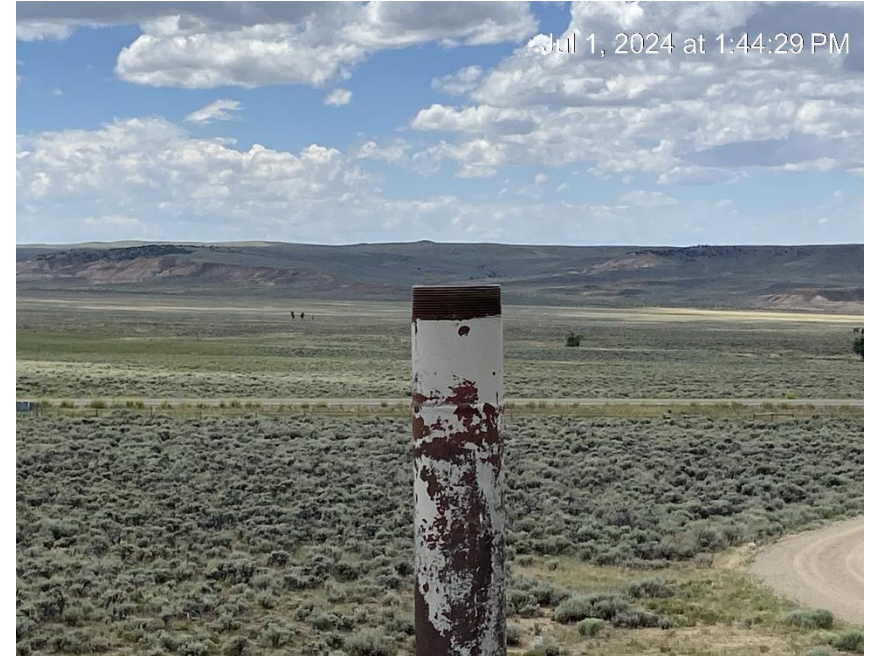
Vent riser missing wildlife protection
