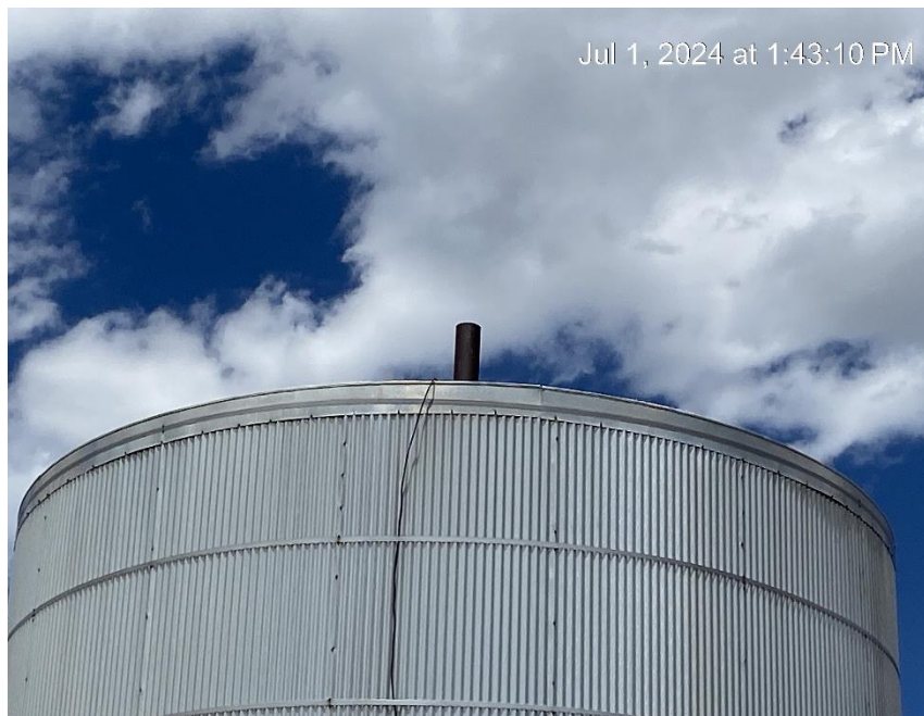
Vent riser missing wildlife protection
