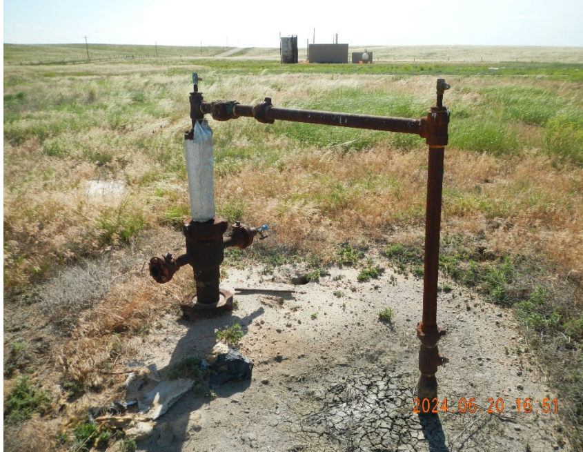
1. View of wellhead. Note vegetation growing across location.
