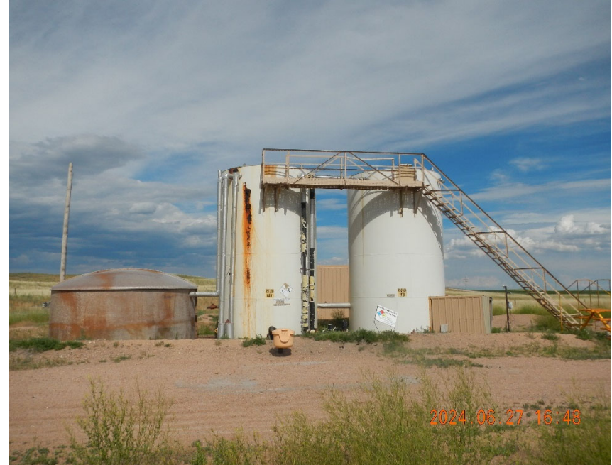
4. View of Tank Battery. Note rust streak down tank on the left.
