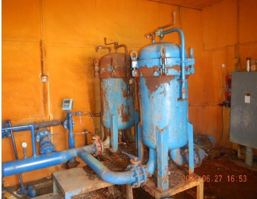
9. View of Filter Pots inside building.
