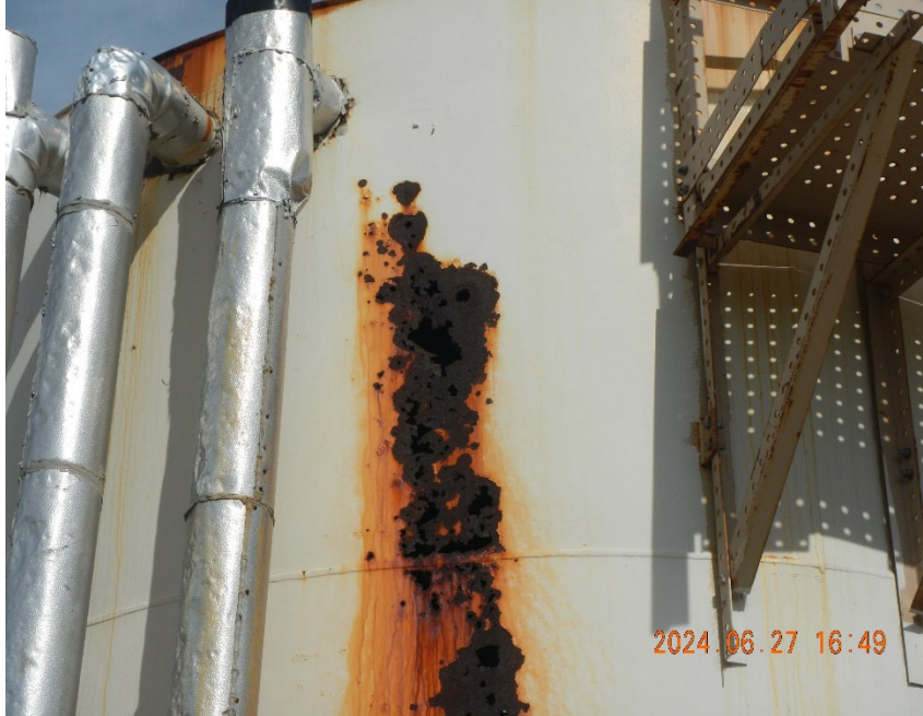
5. Close up of hole in wall of left side 400 BBL tank.
