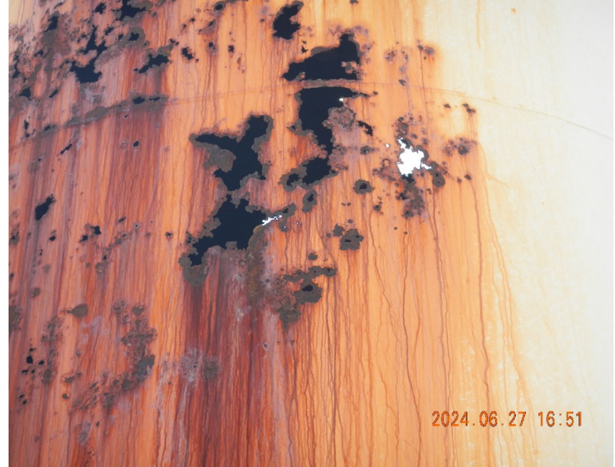
6. Additional view of rusting, holes, and pitting on the backside of the left tanks wall.
