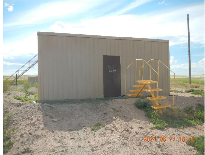
8. Steel Injection Pump and Equipment Building. Note berm has been opened up on left side front of building.
