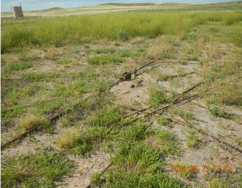
13. Rods and polish rod dumped on location.
