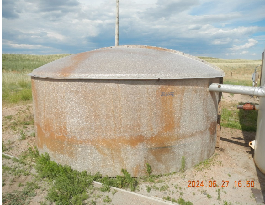
7. View of 200 BBL Tank. No Content/Quantity/Hazard label on tank. Note vegetation.
