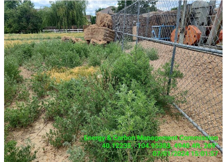
**Photo 5 Large hay bales set as sound damper are degrading falling down and need to be addressed.**
