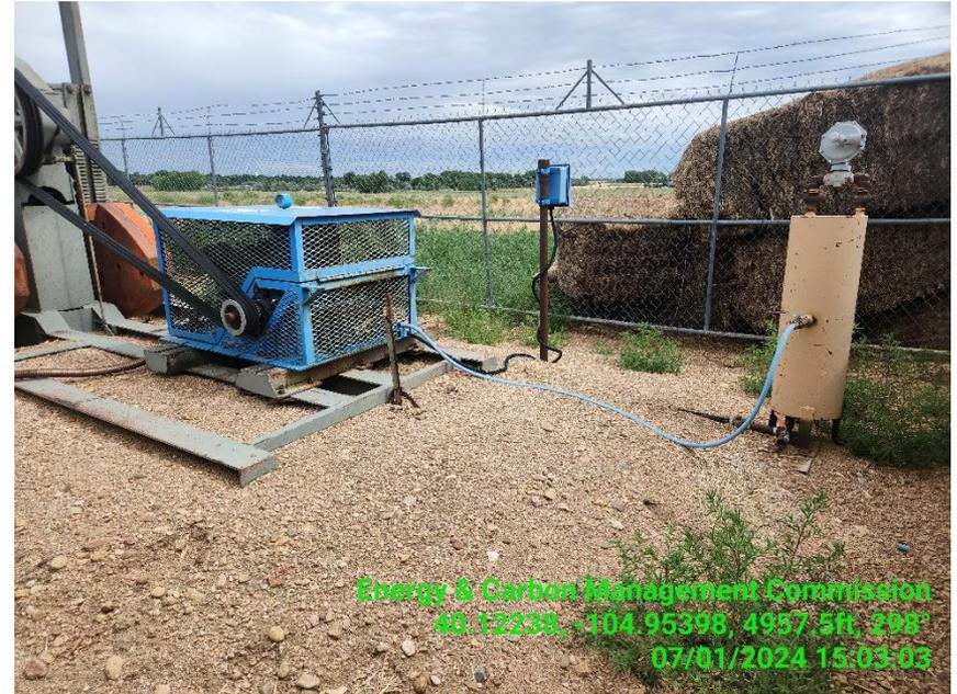
**Photo 9 Large hay bales set as sound damper are degrading, falling down and need to be addressed.**
