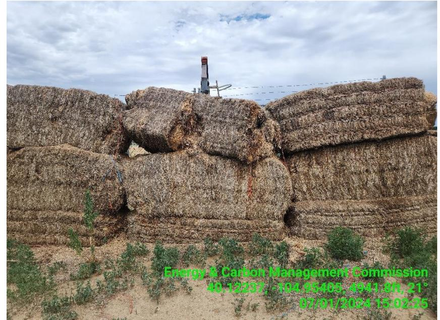
**Photo 7 Large hay bales set as sound damper are degrading, falling down and need to be addressed.**
