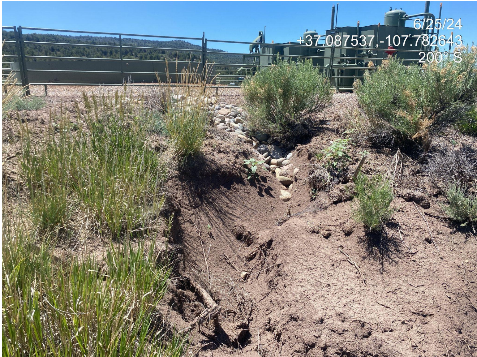
Photo 3. Gully erosion observed forming in the northern interim reclamation area.
