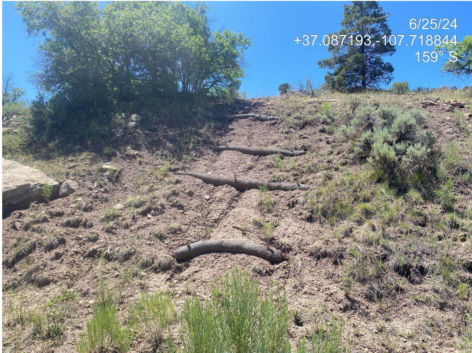
Photo 2. Erosion issues persist in the southern cut slope area. Storm water BMP wattles needs maintenance.
