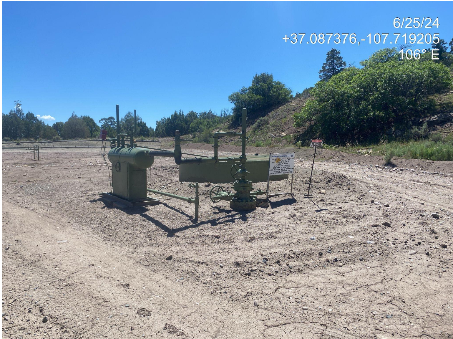
Photo 3. Berm/secondary containment corrective action identified in the previous inspection doc #693903535 has been addressed/resolved.
