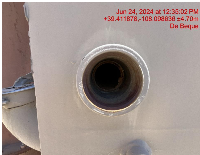
Open ended piping/wildlife hazard - Photo #02890
