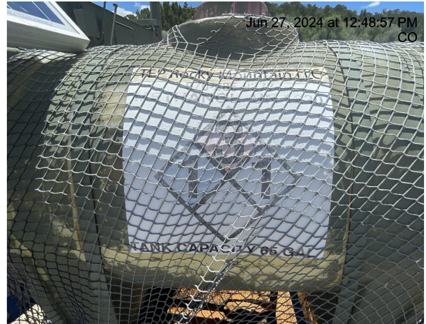
Photo # 1888 Chemical tank label weathered/faded & some required info is illegible
