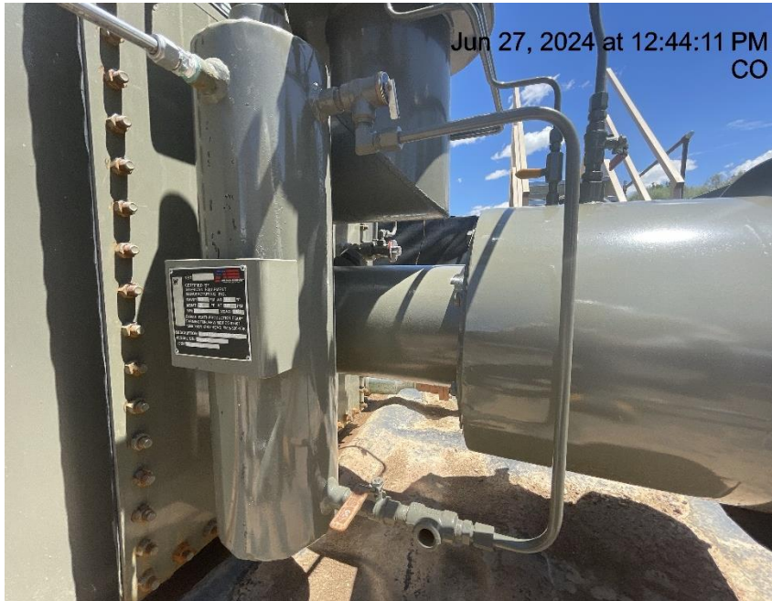
Photo # 1889 PRV vent line does not comply with CECMC pressure safety device rules
