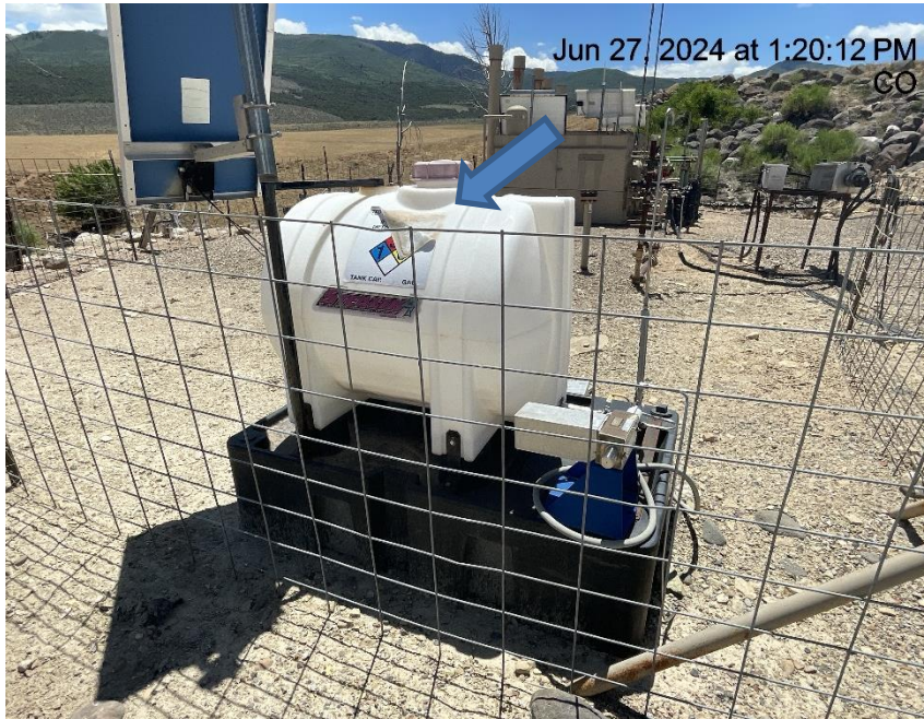
Photo # 1932 Chemical tank label starting to peel & some required info is not visible
