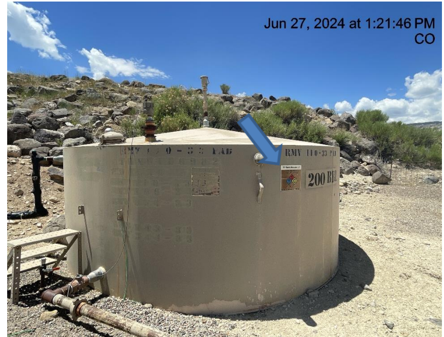
Photo # 1933 Tank label weathered & starting to become illegible
