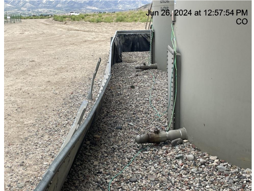
Photo # 1708 Tank containment damaged/buckling
