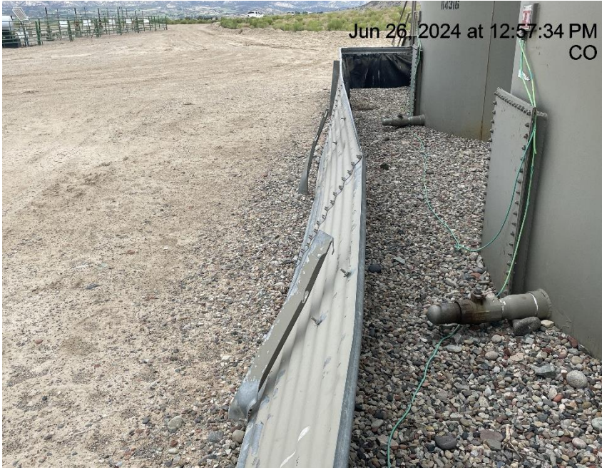
Photo # 1707 Tank containment damaged/buckling
