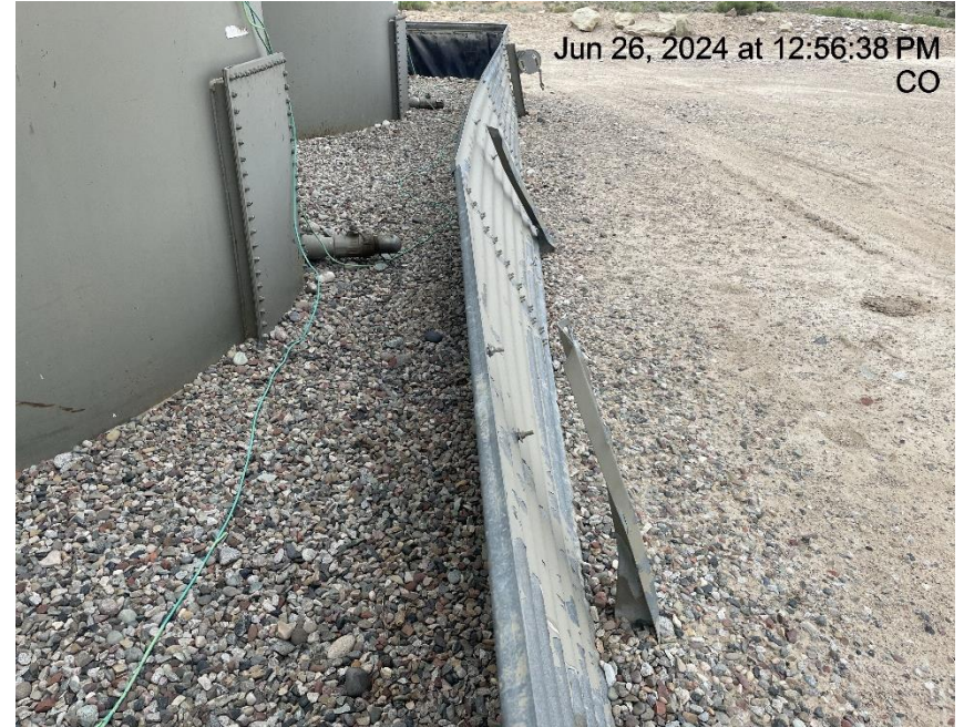
Photo # 1706 Tank containment damaged/buckling
