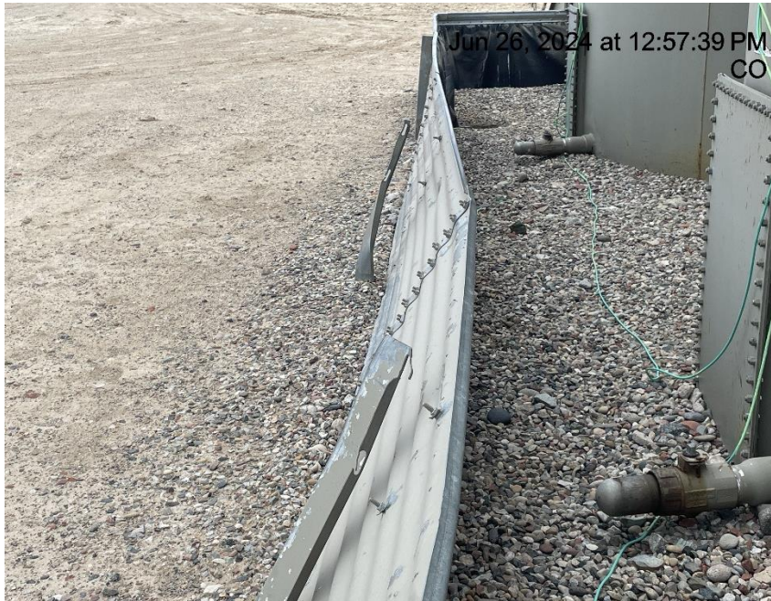
Photo # 1709 Tank containment damaged/buckling
