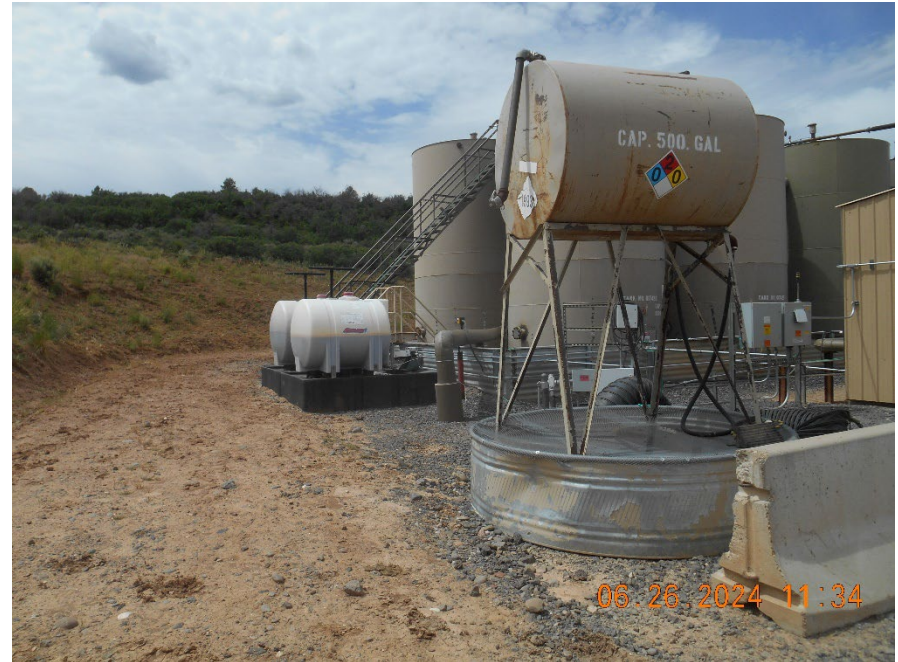
Secondary containment od chemicals
