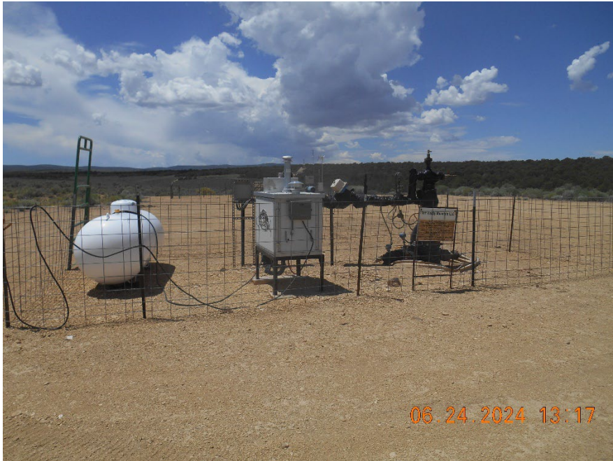
Injection wellhead and line heater
