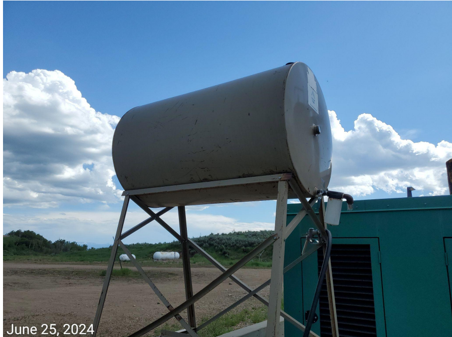
Photo 16: Labels at container no longer legible.
