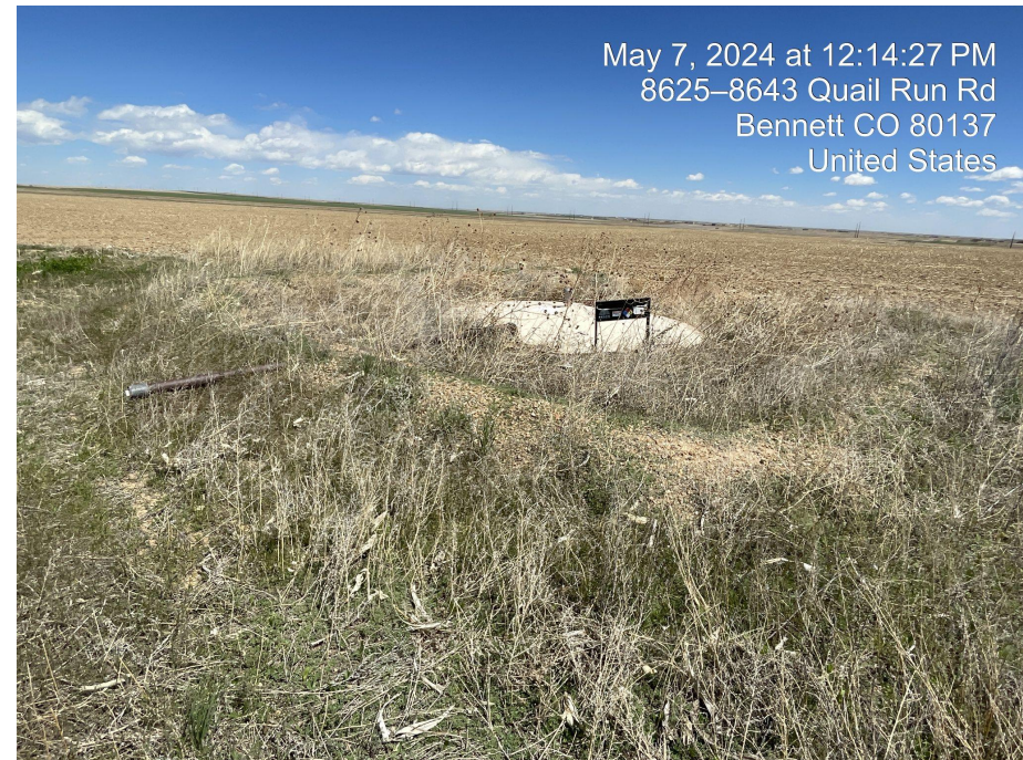
Photo 12. Photo taken facing west of produced water tank in a earthen berm containment covered with weeds.
