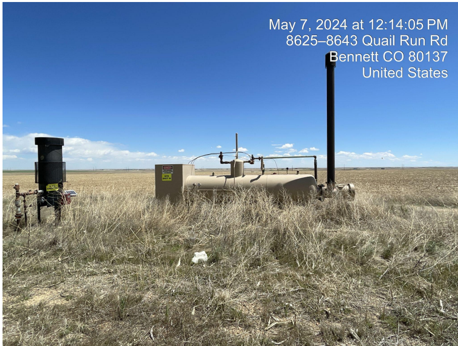
Photo 11. Photo taken facing north of separator and burner surrounded by weeds.
