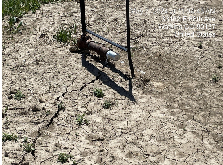
Photo 2. Photo taken of riser on site (the only equipment that could be seen on site).
