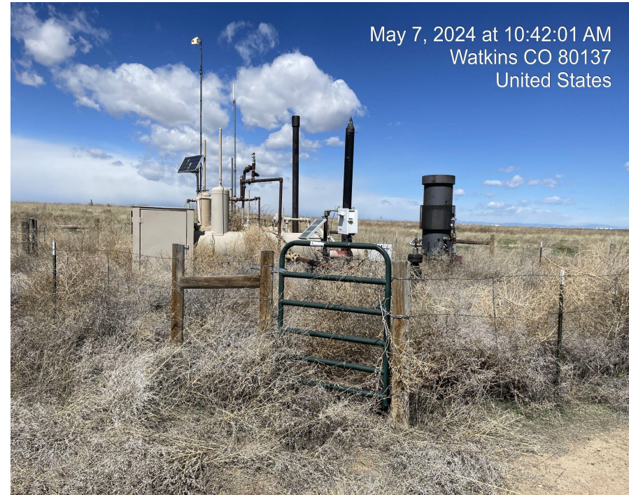
Photo 4. Photo taken facing southeast of burner and separators inundated with weed debris.
