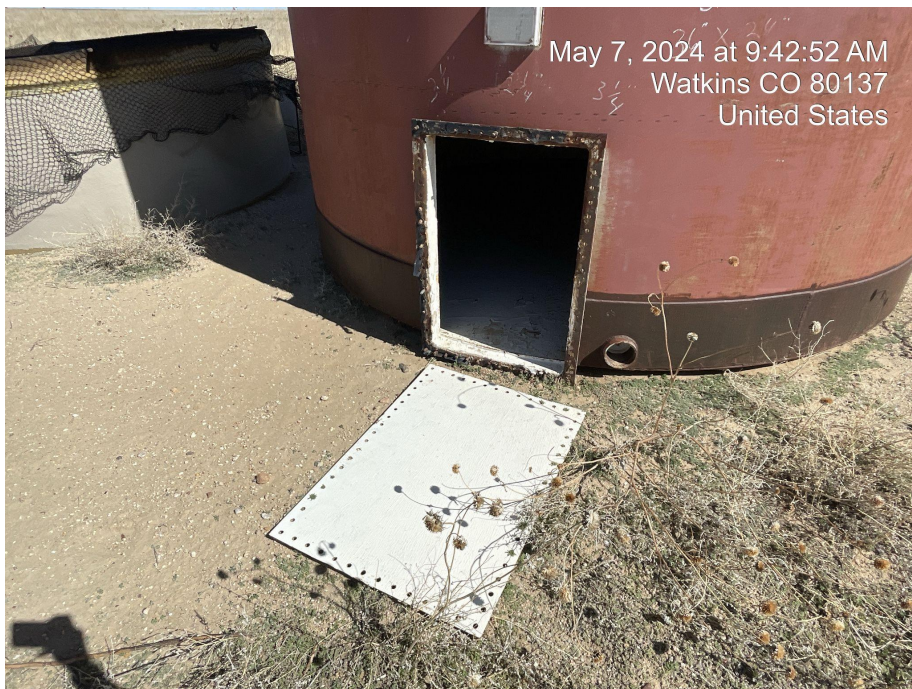
Photo 5. Photo taken of open hatch on empty 300 bbl oil tank.
