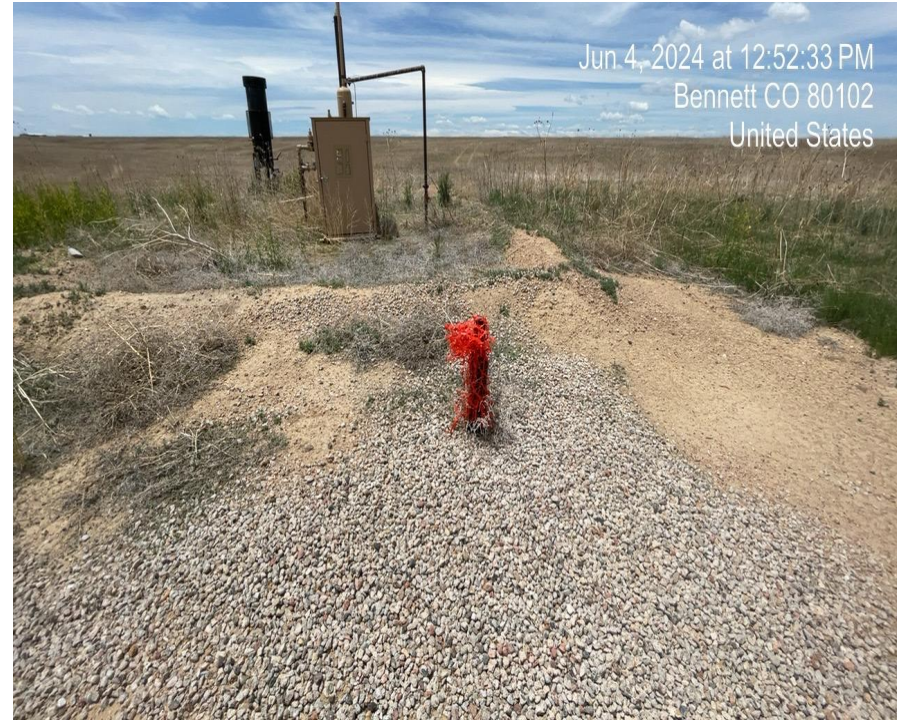
Photo 4. Photo taken facing west of separator and exposed pipe riser.
