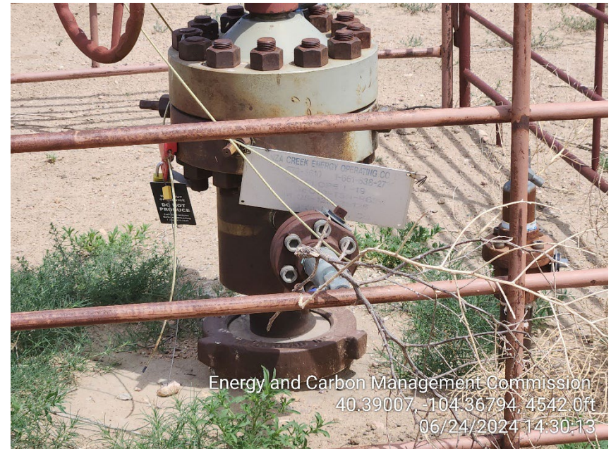
Photo 2 – L-19 Wellhead Sign – Faded no longer visible
