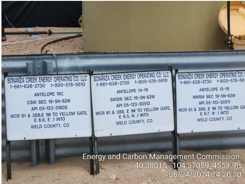
Photo 5 – Tank Battery Signs
