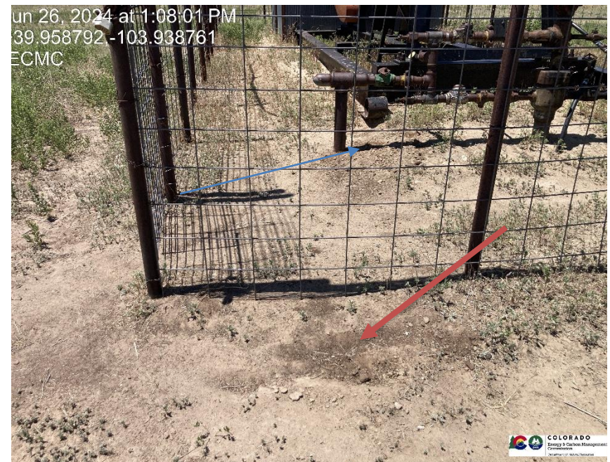
Pic 2 Stained soil was covered by dirt, red arrow shows where dirt was shoveled to cover contaminated soil by wellhead.
