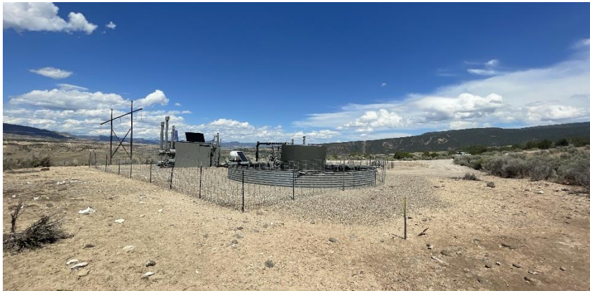
South West corner of location.
