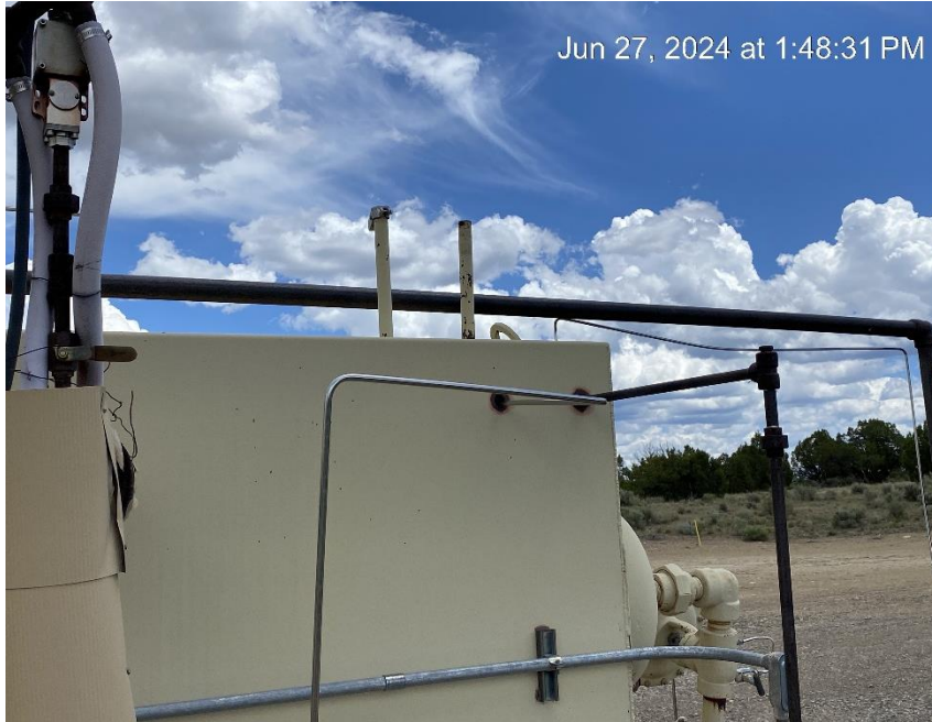
Missing cap on riser
