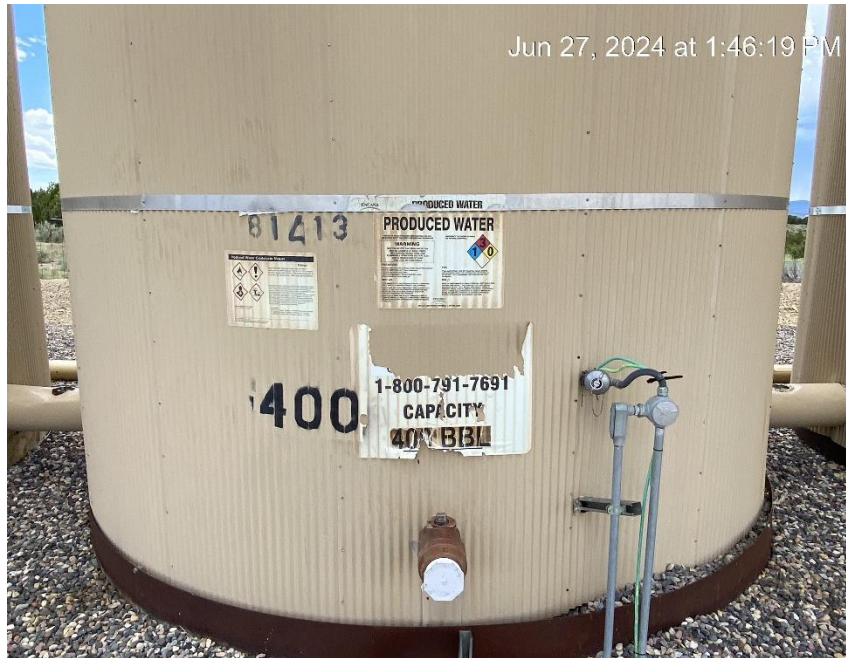
Tank labels incomplete, illegible and/or damaged
