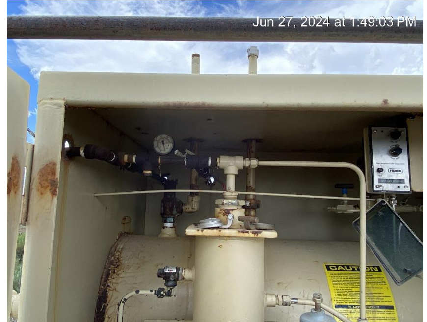
Riser missing protective cap
