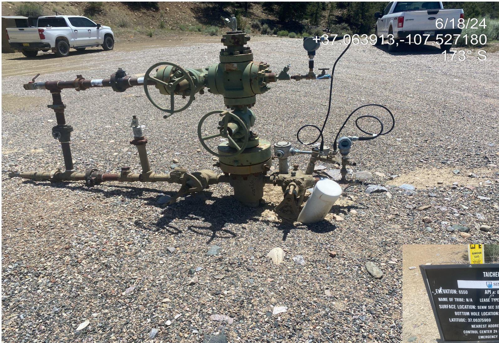
Photo 1. View of the well head assembly taken from the center of the disturbance.
