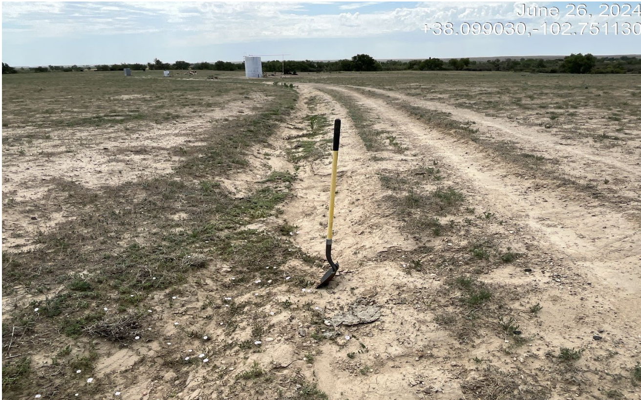
Photo 1. Facing southeast along the access road. There is erosion along the road that must be repaired and stabilized.
