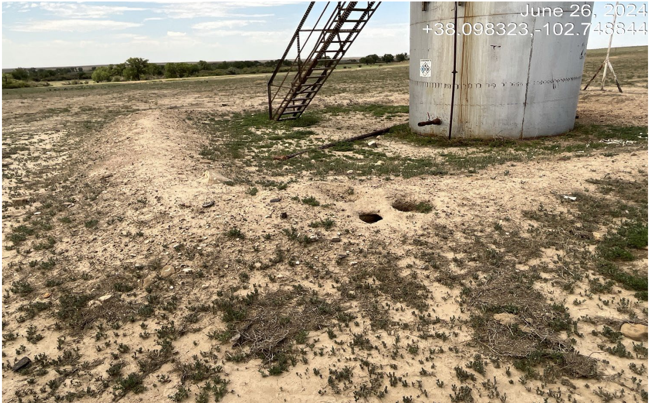
Photo 4. There are holes in the berm which needs maintenance.
