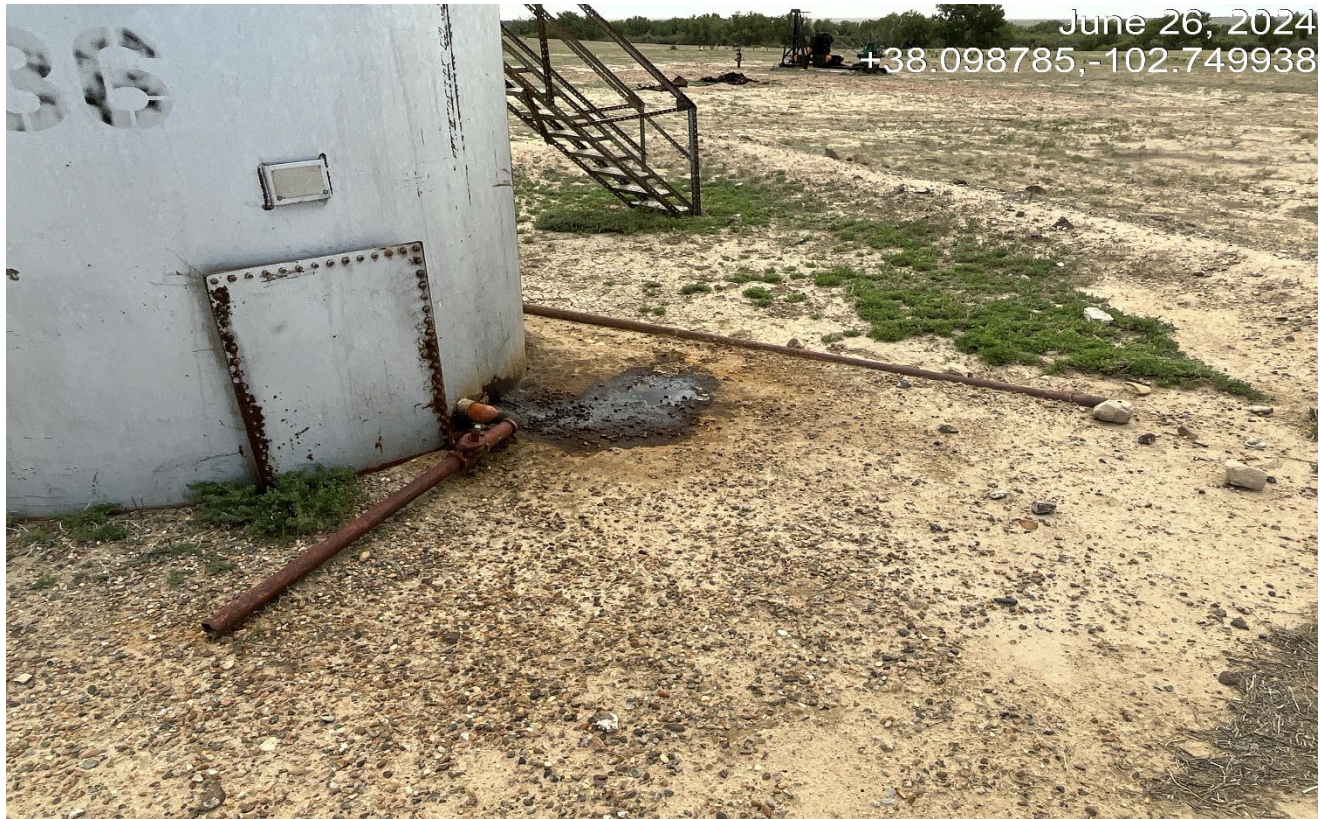
Photo 3. There is an oil leak by the outlet that needs to be controlled and cleaned up!
