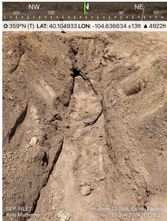
Separator Inlet Excavation
