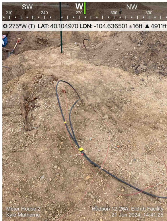
Meter House Excavation
