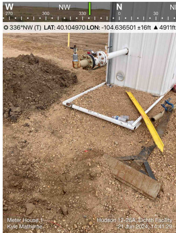
Meter House Sample Location
