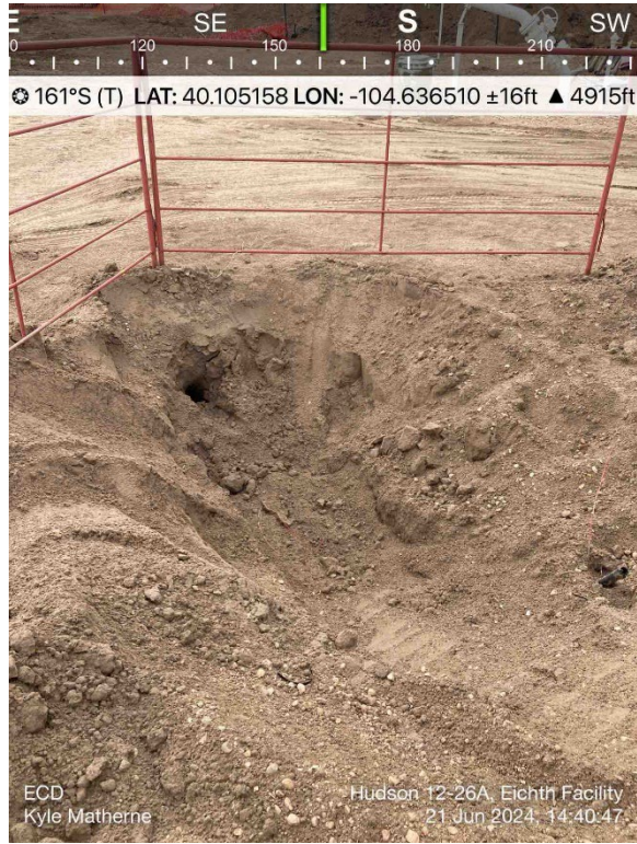
Emission Control Device (ECD) Excavation
