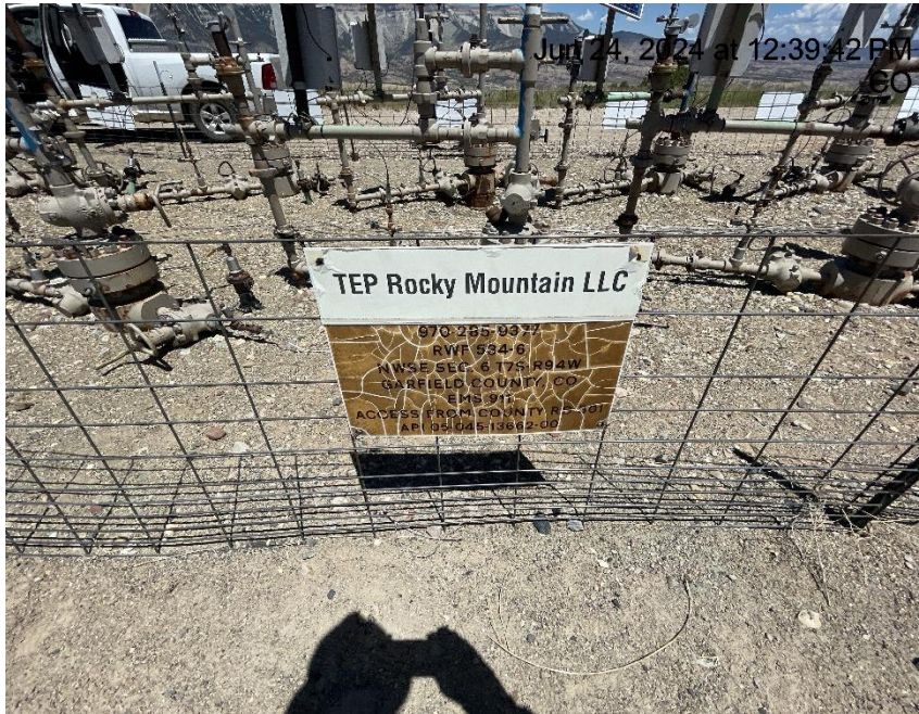
Photo # 1292 Wellhead sign weathered & cracking/starting to become illegible
