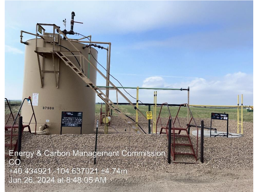
Photo 4 Tank Battery
