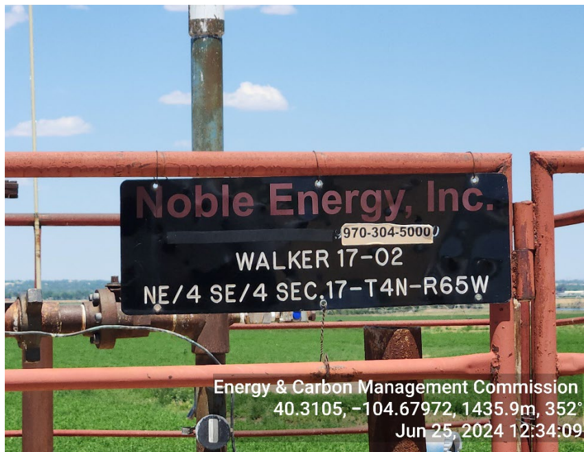
Photo 1: Wellhead Sign; incorrect wellhead name
