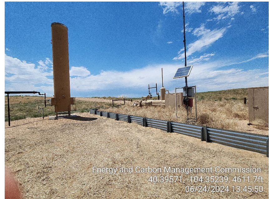
Photo 12 – ECD and Separator – Tumbleweeds
