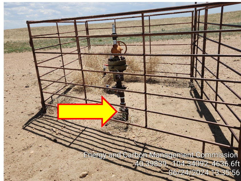
Photo 8 – Unmarked 1" Riser
