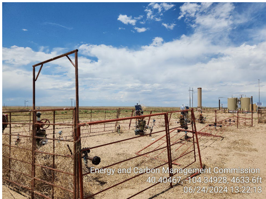
Photo 3 – Wellheads – Panels in disrepair
