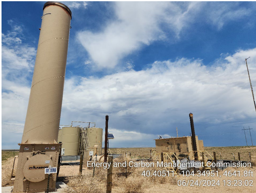
Photo 5 – Separators and ECD – Tumbleweeds
