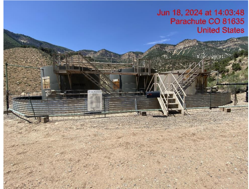
Tank Battery – Photo #01813
