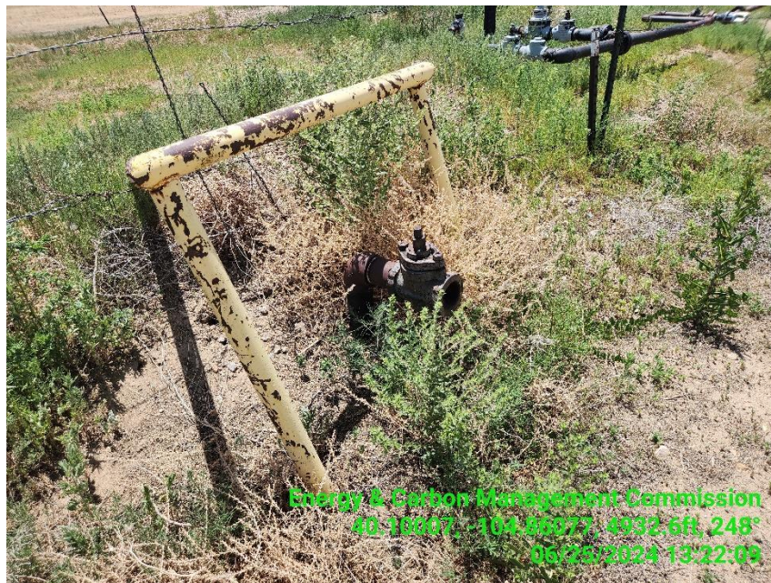
Photo 7 Flow line valve North of the TB.
