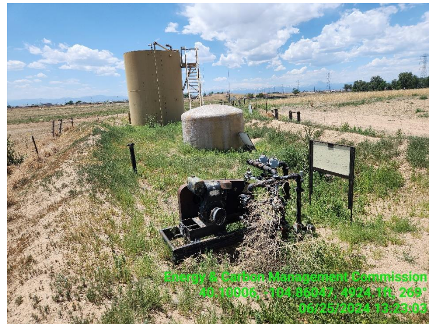
Photo 10 Tank battery, flow line manifold & aux pump.
