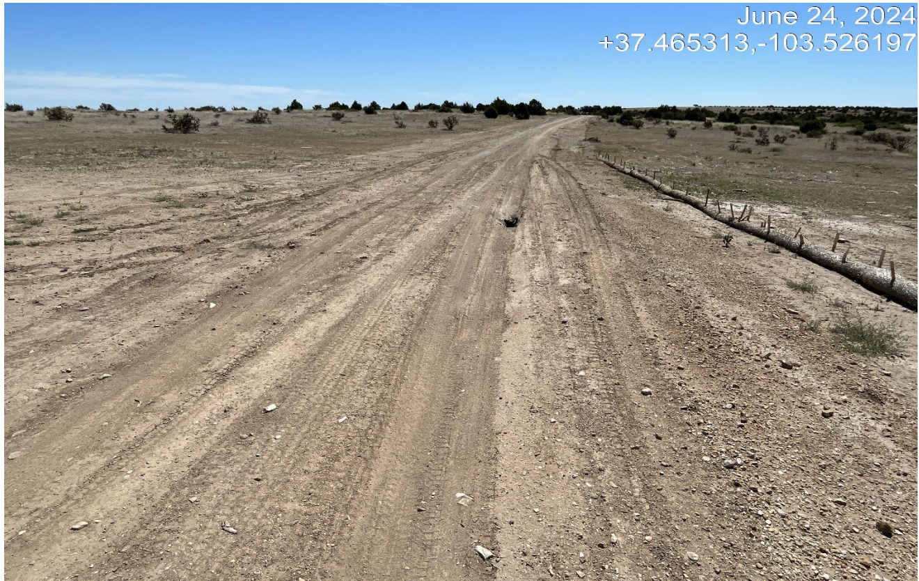
Photo 3. Facing east toward the flowline disturbance. The vegetation is not establishing along the flowline and there are vehicle tracks which are causing unnecessary disturbance. The flowline must be reclaimed and stabilized.
