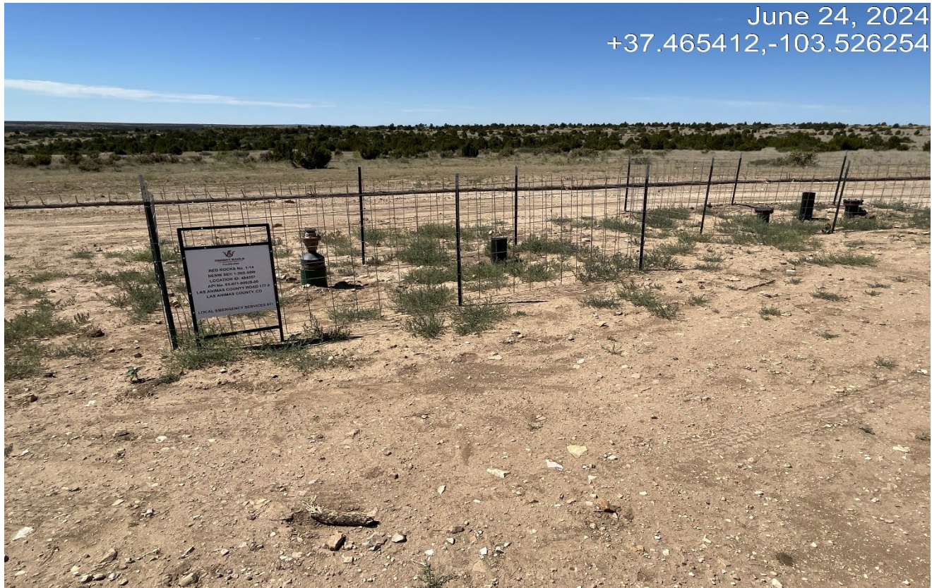
Photo 2. Facing east toward along the access road near the location. There are area where soils are very compacted. Seeding was performed in this area however vegetation will not grow well in compacted soils.
