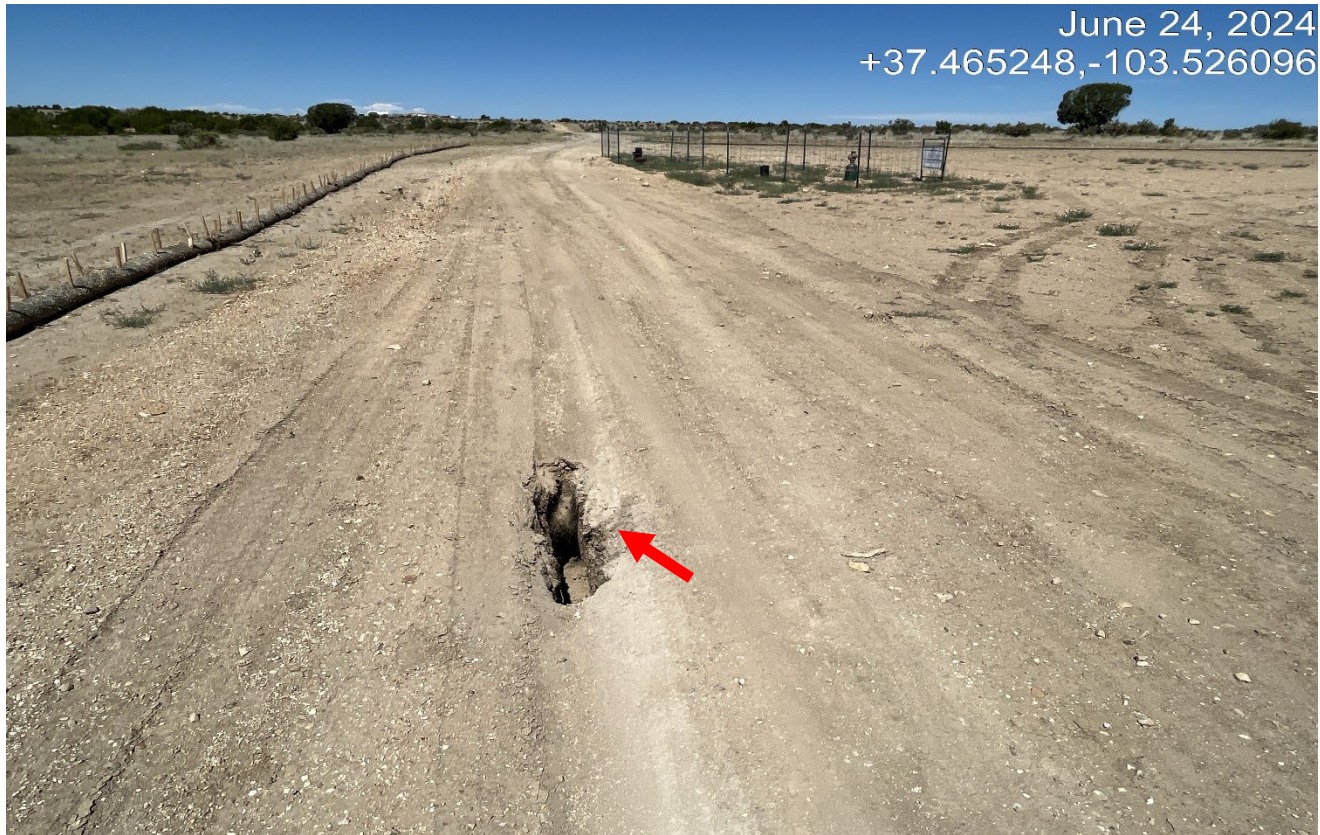
Photo 4. Facing west toward the flowline disturbance. There is an area of subsidence that needs to be filled in.
