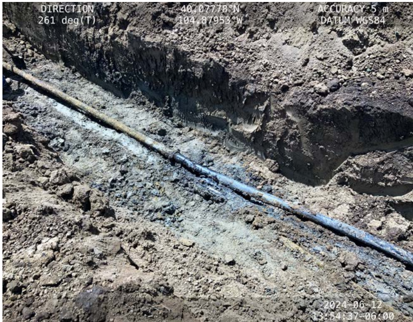
Photo 9 – Stained soil within the excavation. Release point
