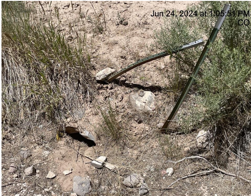
Photo # 1315 Sediment buildup in culvert & capacity has been reduced, may need maintenance in the near future (Near entrance to location)
