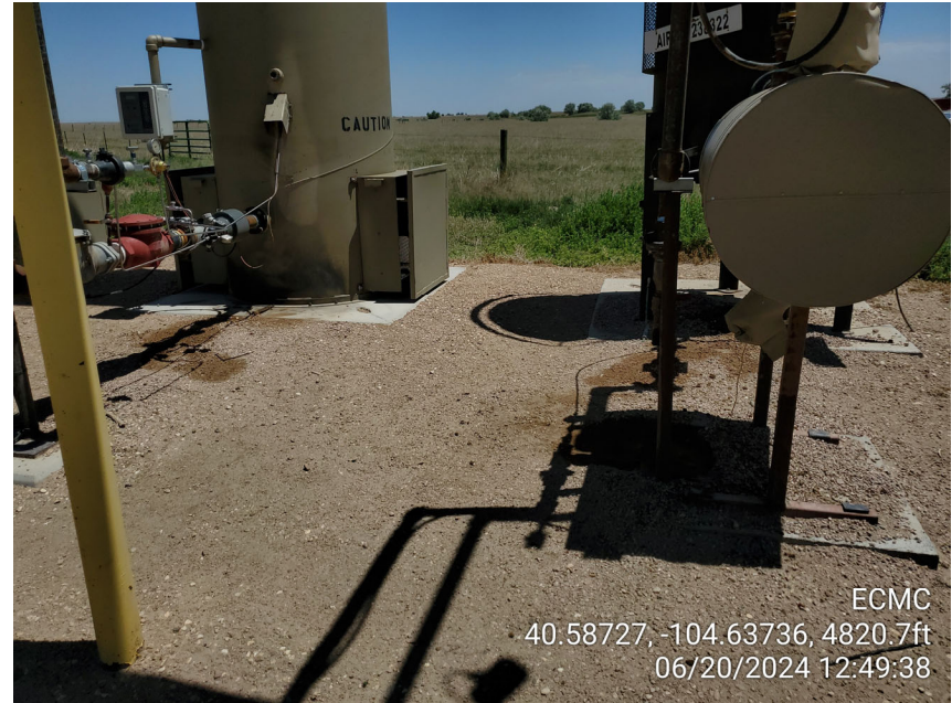
Photo 4 Spills around Emission Control Devices
