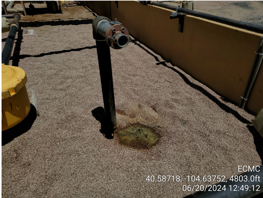
Photo 3 Spill at riser within tank battery secondary containment
