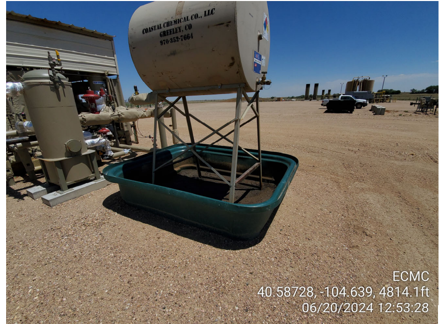
Photo 6 Secondary containment around chemical tank lacks wildlife BMPs
