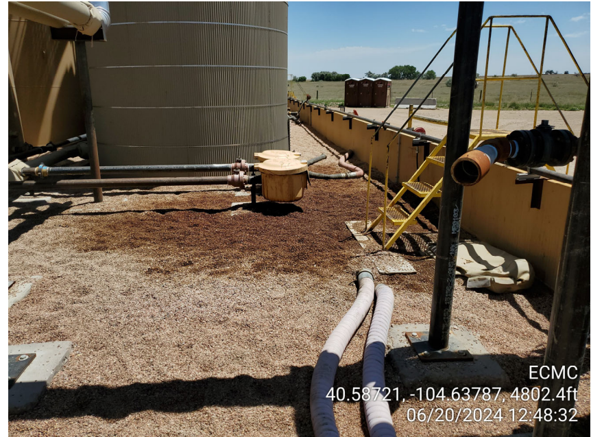
Photo 2 Spills within tank battery secondary containment
