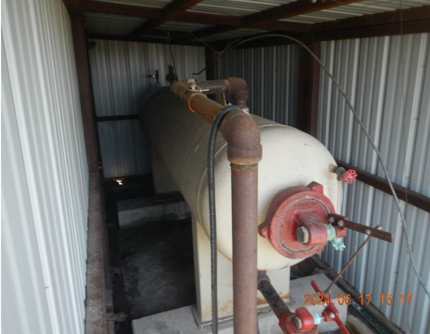
3. Horizontal separator inside separator shed.
