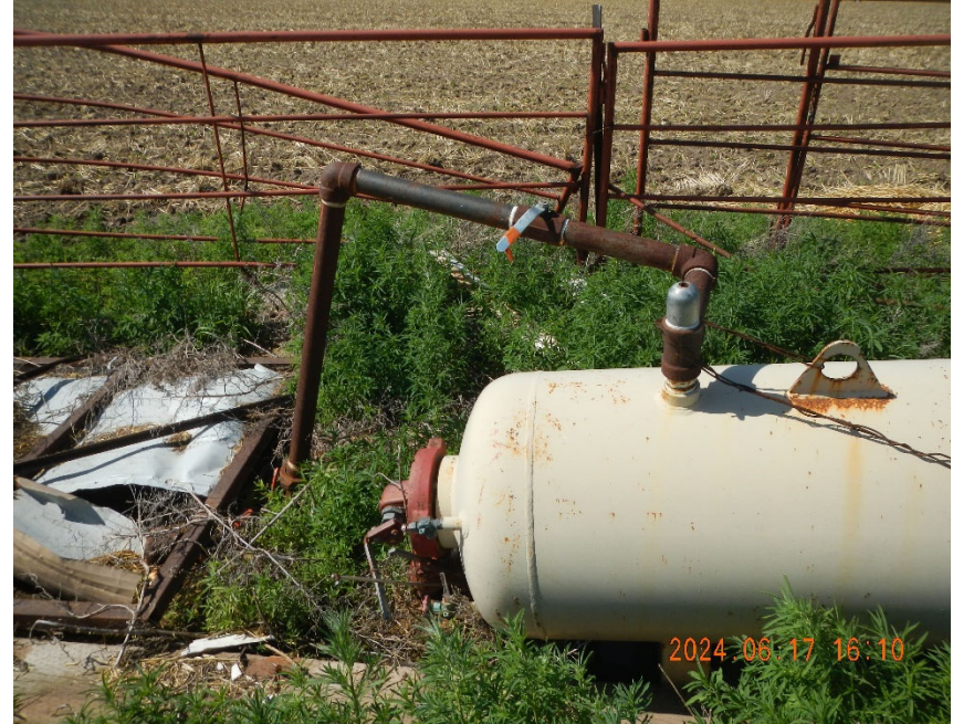
4. Flowline out of separator.
