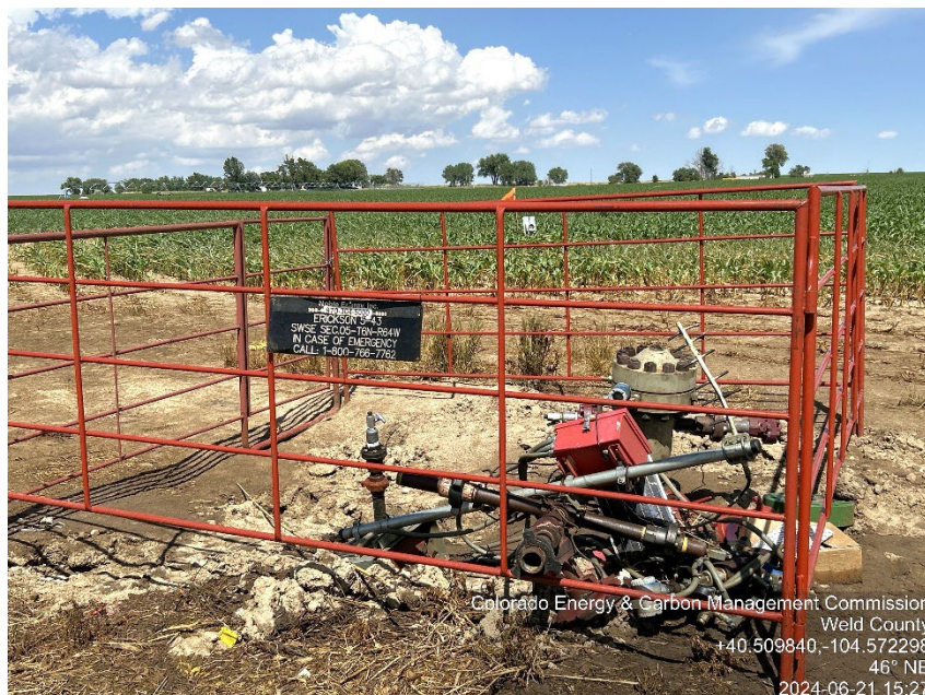
Photo #3 Erickson 5-43 Wellsite Temporarily Abandoned | TA Incident: WH strike; 2024-06-14
