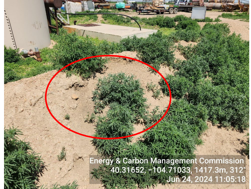
Photo 10: weeds, damaged berm
