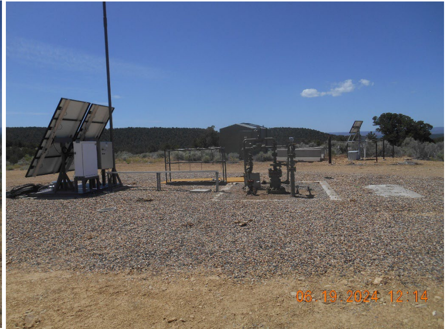
Injection Wellhead
