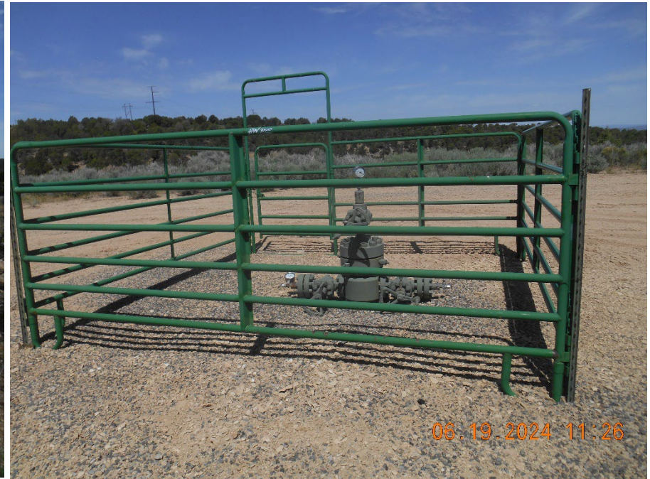
Injection Wellhead
